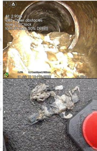
Images - partial blockages proactively identified and resolved through DNM.
